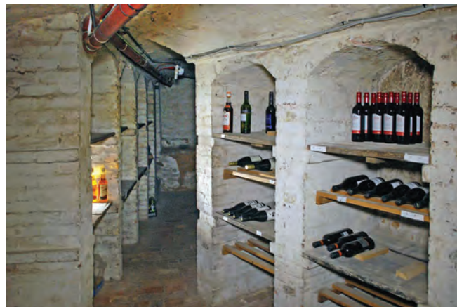
Unusually for a Dorking inn all the wine bays are neatly finished in brick
